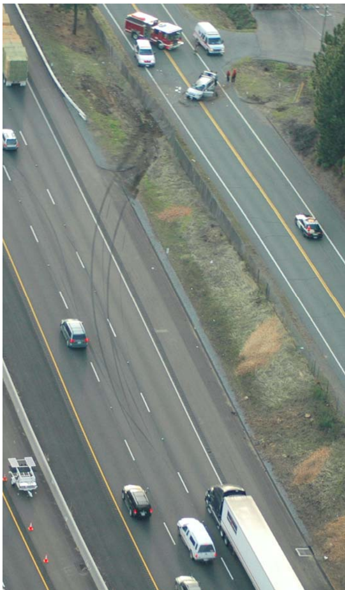
Tread marks scarring highway asphalt reveal the story of a dramatic crash event.
